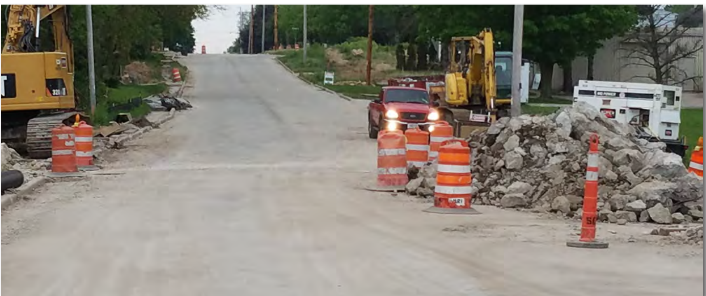
Maple Avenue Reconstruction
