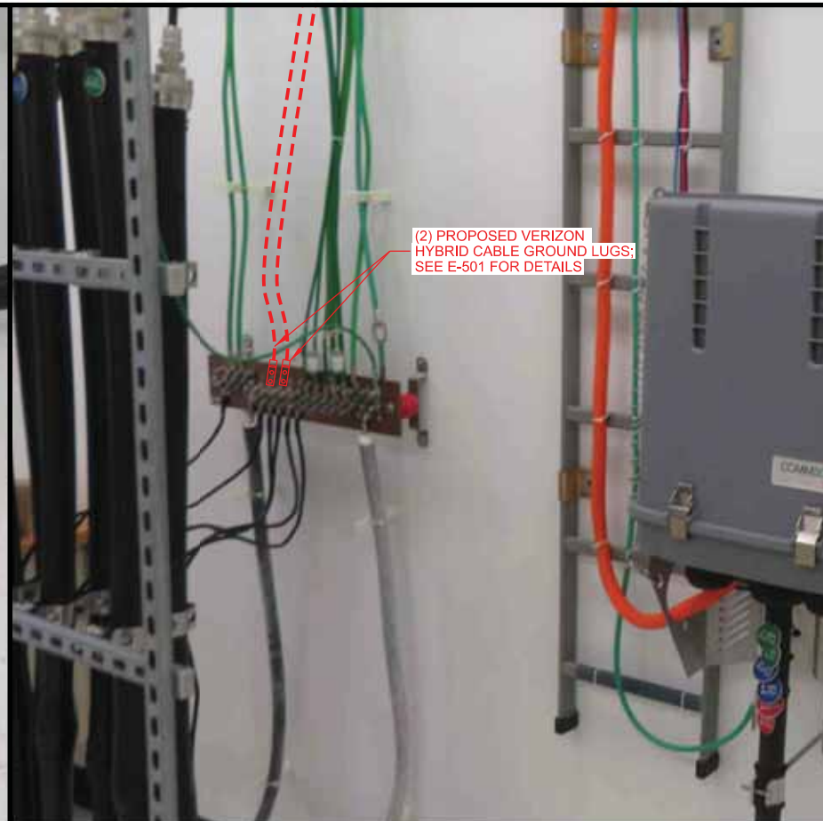
B SHELTER GROUND BAR (SHELTER INTERIOR)
