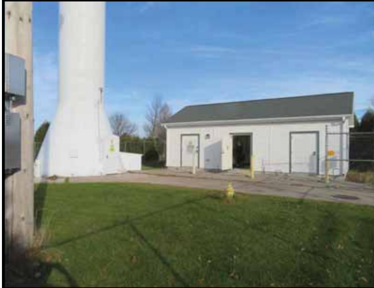
B COMPOUND OVERVIEW
