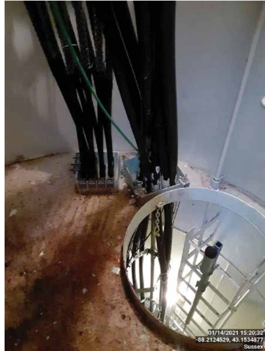
PHOTO OF SAFETY CLIMB
