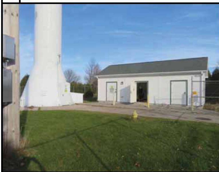
B COMPOUND OVERVIEW
