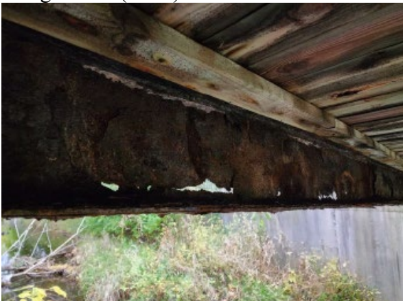
Bridge beam (north) after removal of scale
