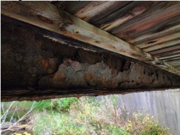
Bridge beam (north) after removal of scale
