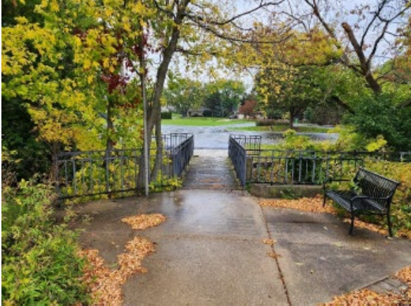
Bridge Beam (north) before removal of scale.
