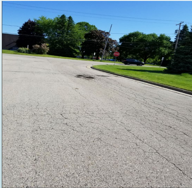
Photo 3: Hi-Tech Drive Pavement
