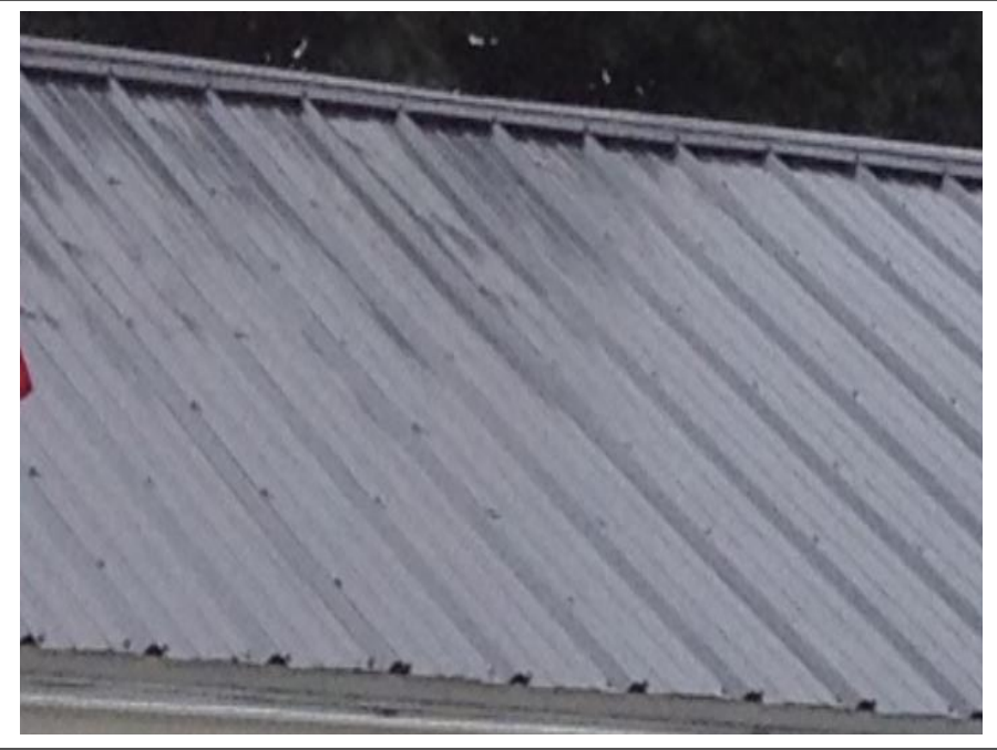
Exposed fastener metal roof system
