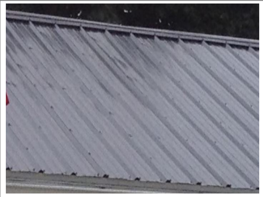
Exposed fastener metal roof system
