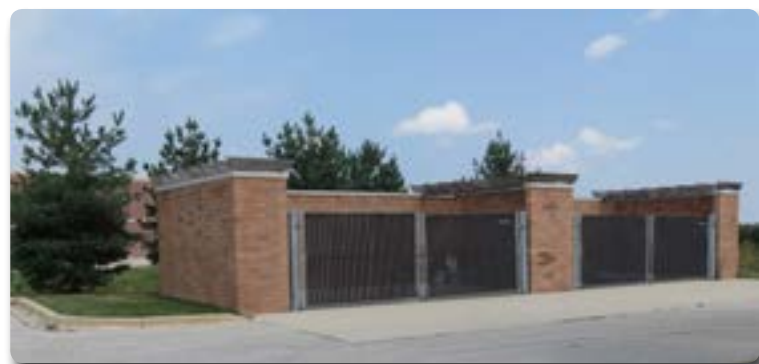
Example of refuse structure designed to blend with the overall site.
