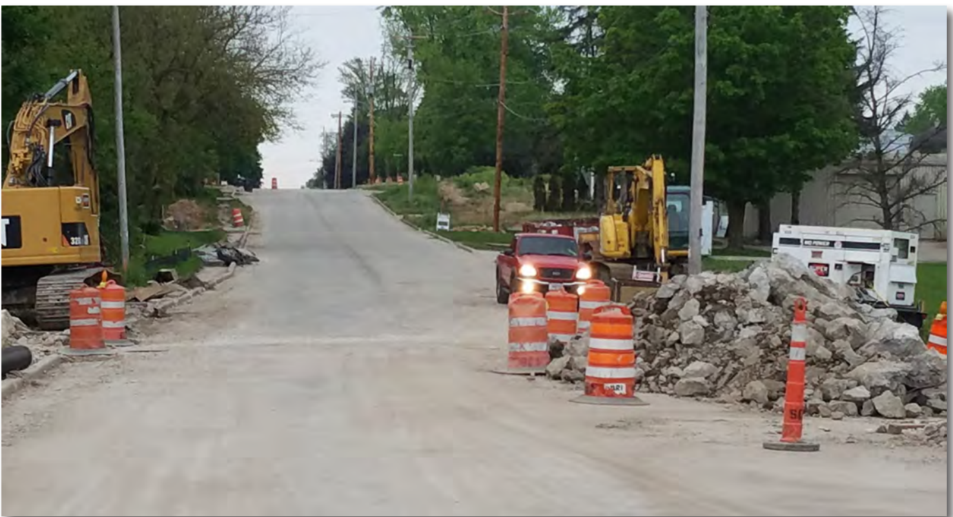
Maple Avenue Reconstruction
